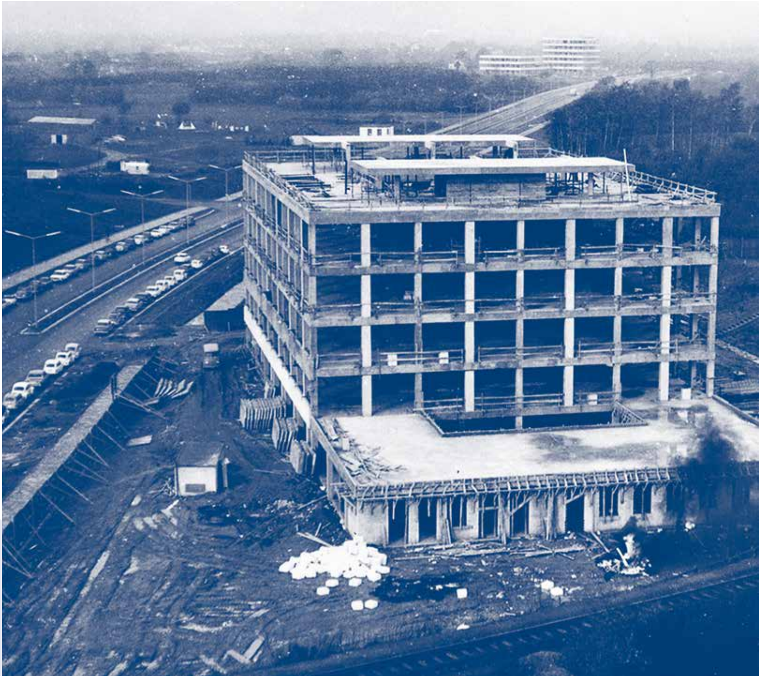
The IPN building under construction around 1969.
